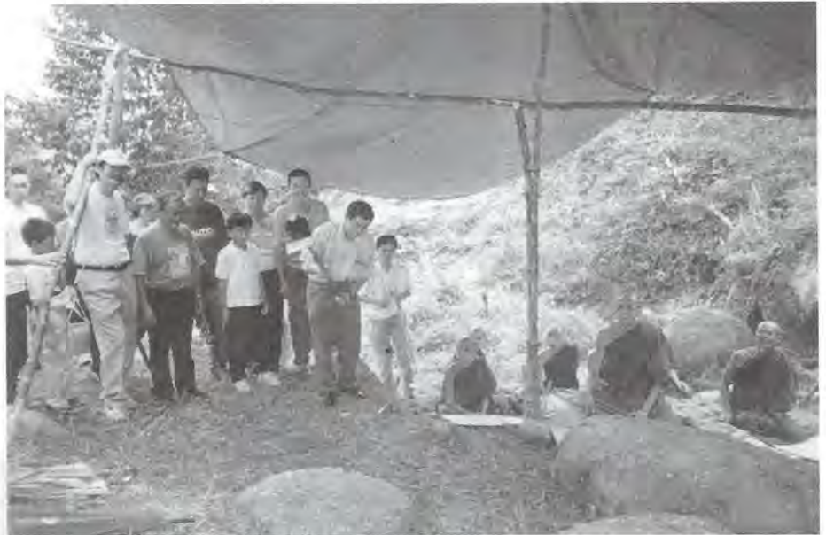
NOT JUST CANGKUL ANGIN... YB Ho breaks the ground at the spot where the boulders will eventually be blasted.
